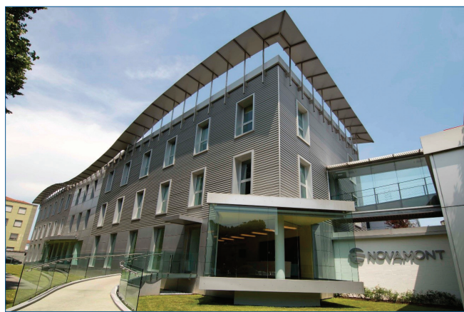
Novamont Headquarter and Research Center - Novara, Piedmont
